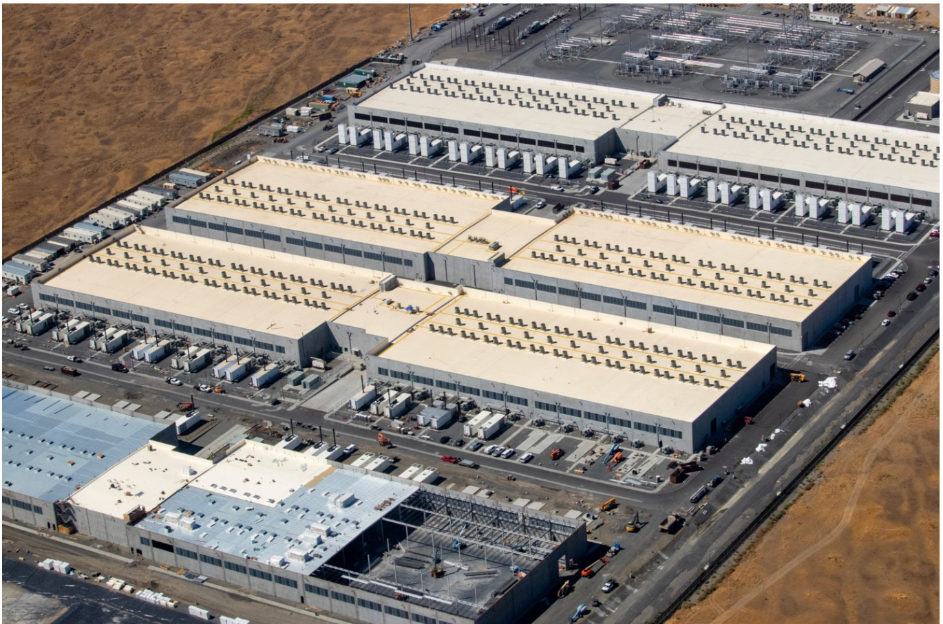
AWS Expanding Data Center, Boardman, Oregon, 2023. Source: Tedder
