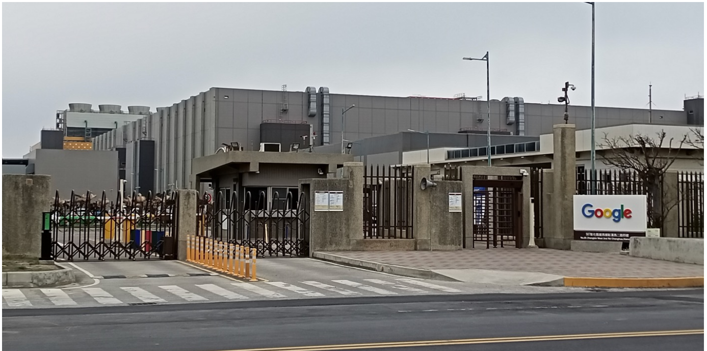
Exterior view of the main gate, Google's Taiwan data center in Xianxi, Changhua, 7 March 2021, cropped top and bottom. Source: Kai3952 .
